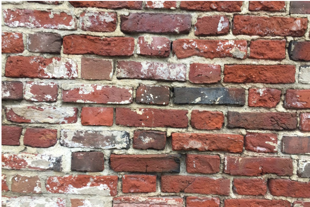
Figure 2. Presumed original wall brick work, with eroded bricks and eroded lime mortar joints.
