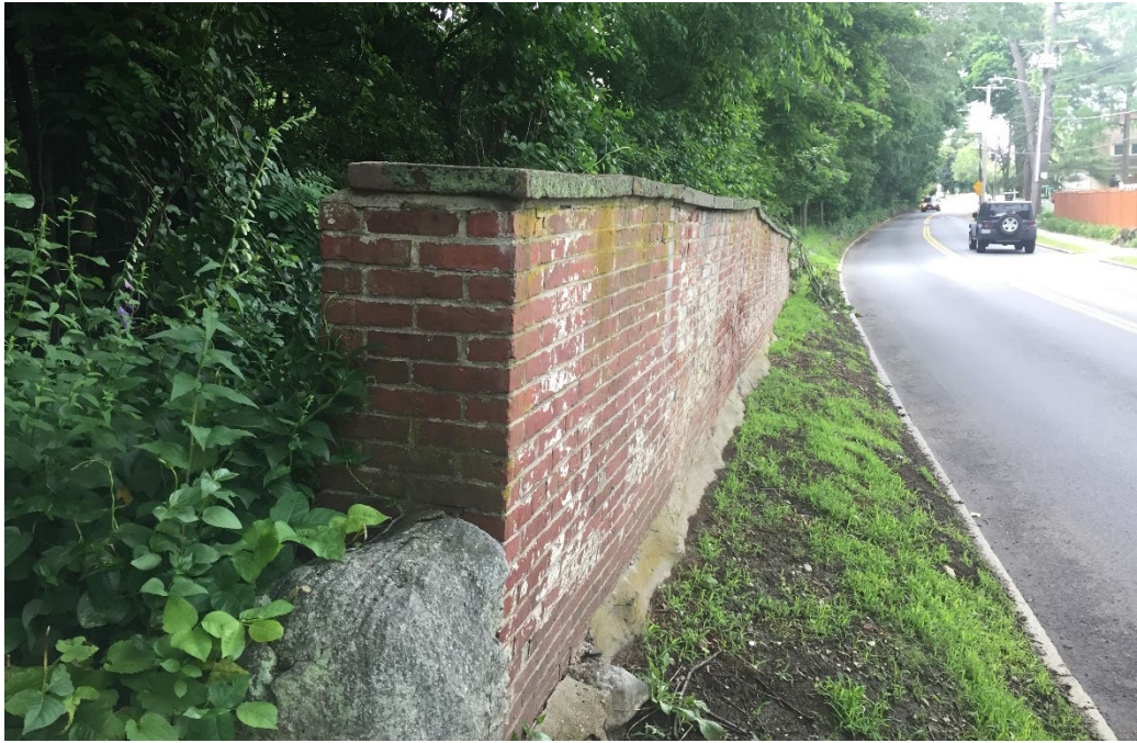
Figure 5. North end of wall – out of plumb and leaning towards road.
