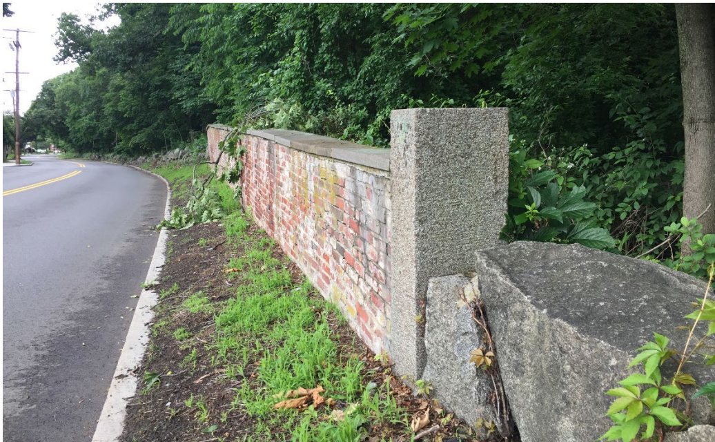
Figure 6. South end of wall – nearly plumb – with soil built up against wall footer.
