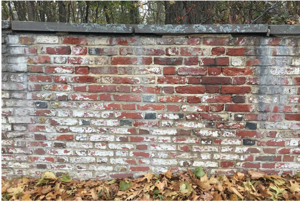
Figure 1. Typical wall condition mid-wall.
