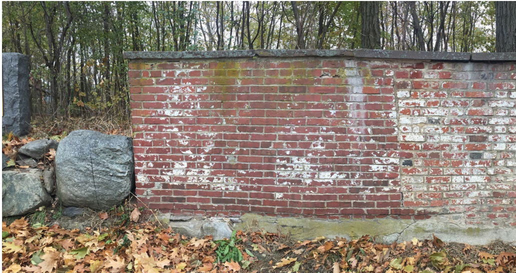
Figure 3. North end of wall – presumably added late 19 th century – with vertical joint separation.
