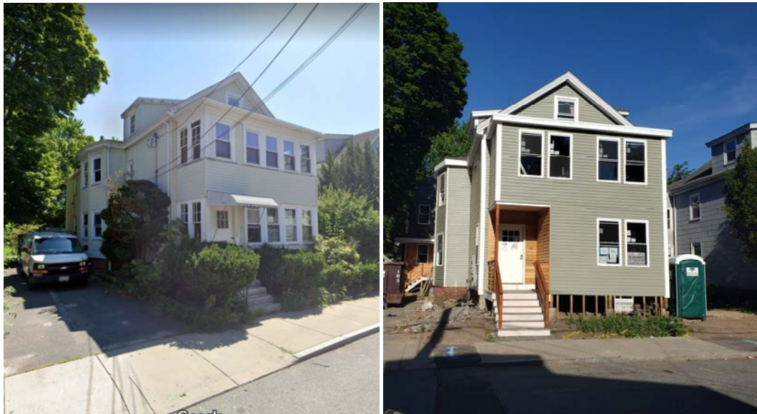
Figure 6 - 277 Park Street before and after demolition. Note the existing front porch was entirely demolished and architectural plans call for them to be open. The owner infilled as shown.
