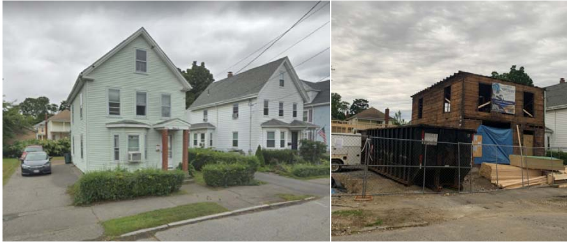
Figure 1 – 22 West Street before and after demolition. The removal of the front bay, roof, siding and interior finishes constitutes substantial demolition and is reviewable under the demolition delay ordinance.
