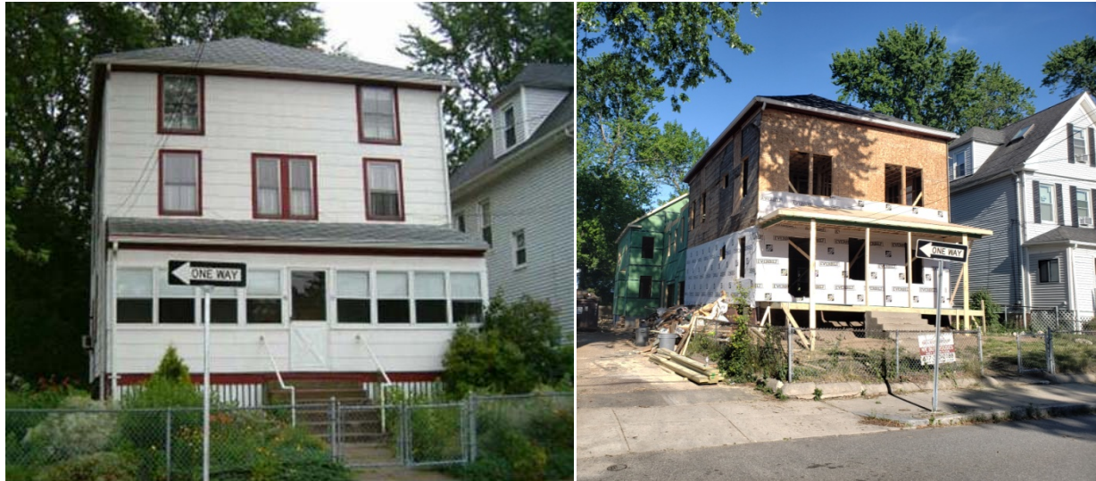
Figure 7 - 77 Court Street under construction. The third level has been entirely removed although the massing has remained the same. A rear addition is under way.
