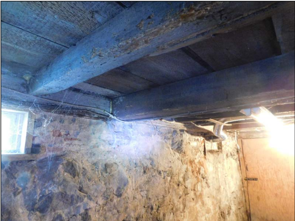
Cellar: hand-hewn joists and sill.
