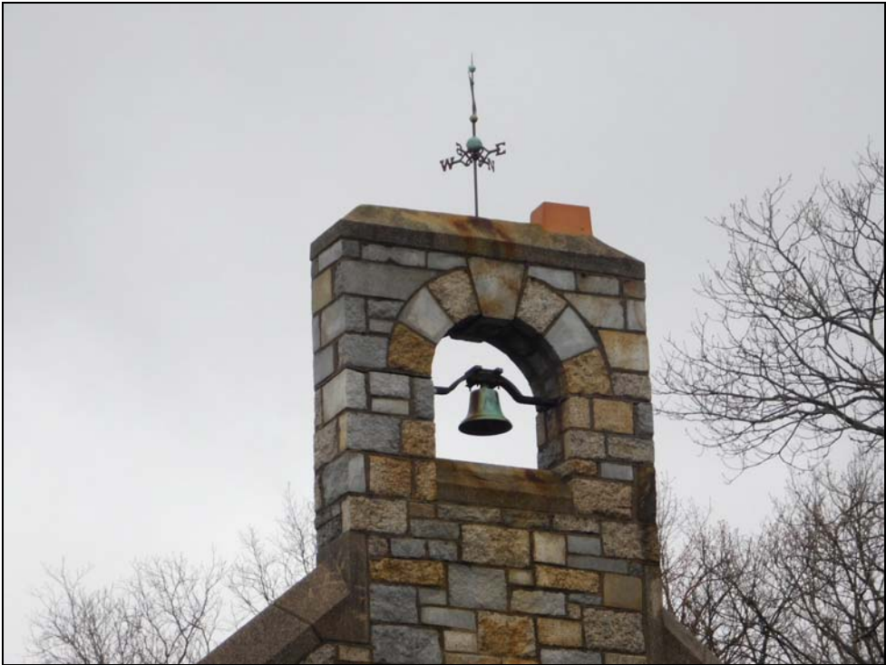
Detail of belfry and granite coping from E.
