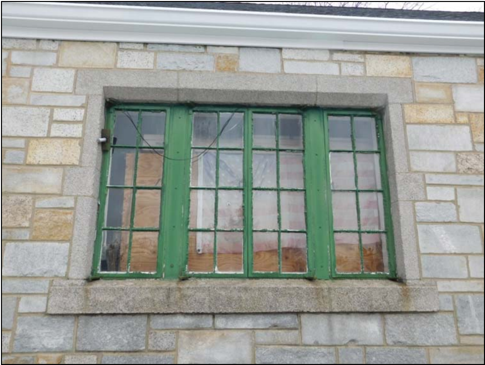
Detail of windows in the façade of the left (west) wing showing rolled steel casement windows, stone casings and mullions.
