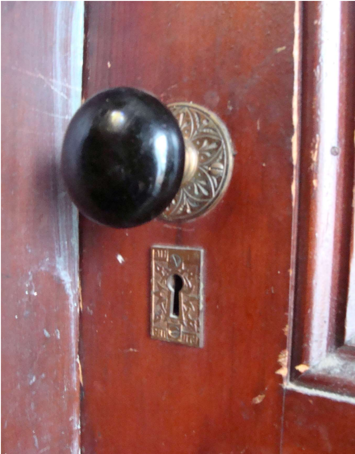
Figure 10. Detail, doorknob and bronze knob and lock escutcheon plates with geometric patterns are found on all of the doors in the house. December 2015. Photograph by Myron O. Stachiw.
