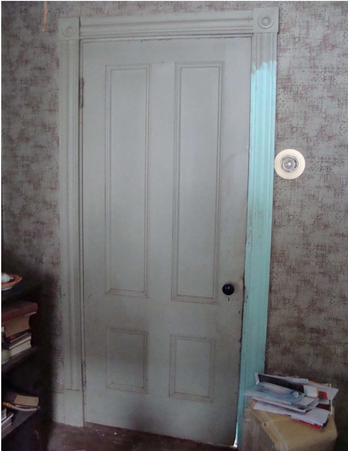
Figure 11. Doorway from the parlor (Rm. 102) to the front entry stair hall (Rm. 101). All of the doorways in Rms. 101, 102, and 104 are trimmed with the same molded architraves with bull's eye corner blocks. December 2015. Photograph by Myron O. Stachiw.
