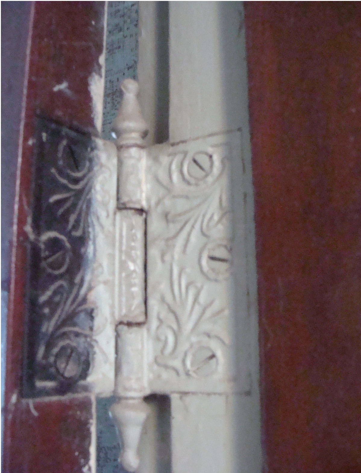
Figure 9. Detail, cast bronze hinges with a floral pattern are found throughout the house on all of the doors. December 2015. Photograph by Myron O. Stachiw.
