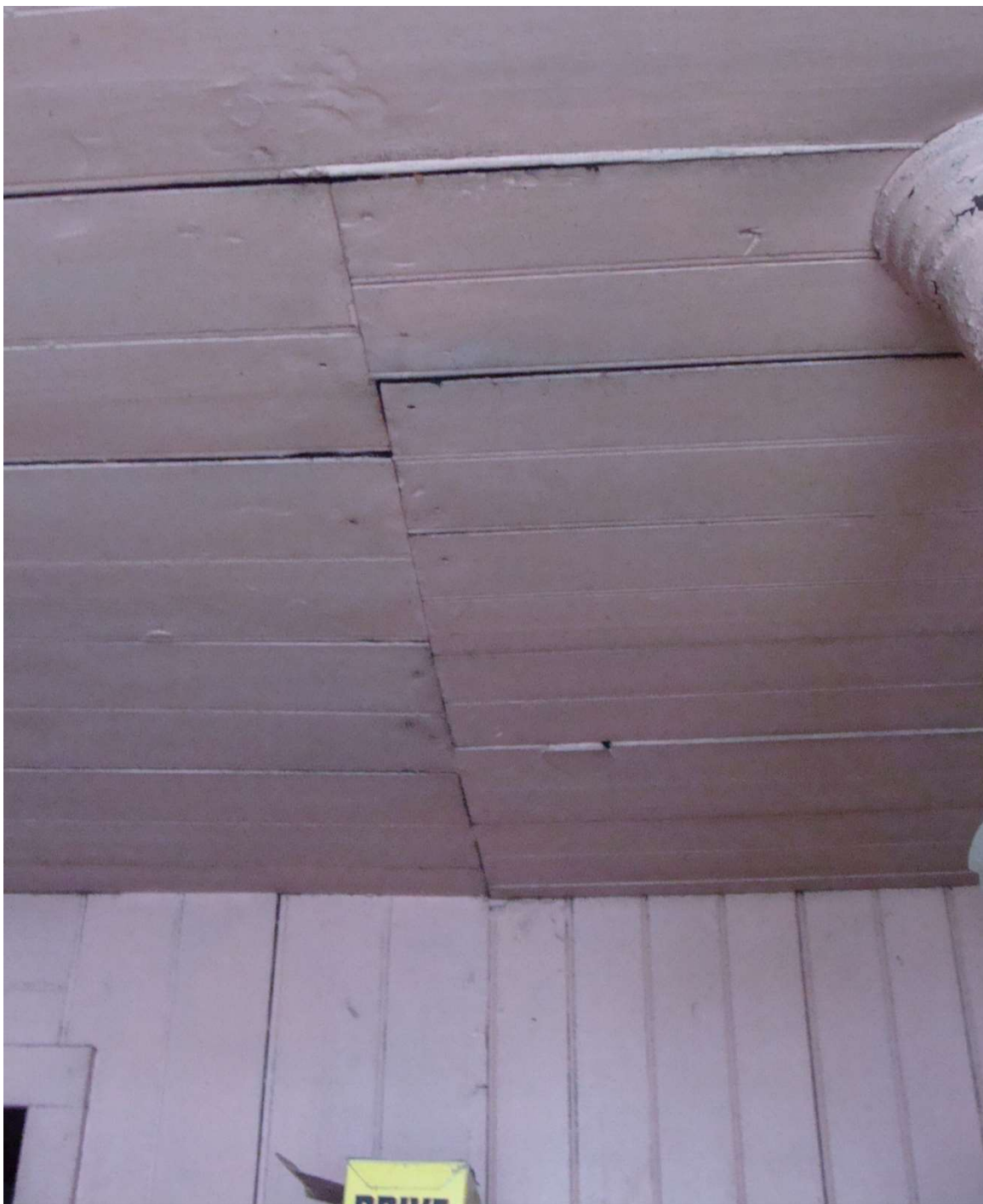
Figure 5. View of patched-in area of the ceiling (to the right of the seam) of Rm. 105 in the rear ell indicating the location of the original staircase to the cellar. At lower left of the image is the corner of the doorway into Rm. 106 in the southeast corner of the rear ell. Looking south. December 2015. Photograph by Myron O. Stachiw.
