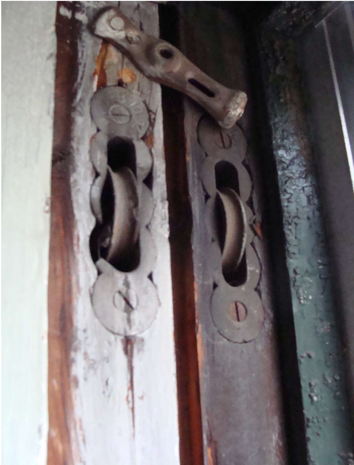
Figure 14. Detail, sash pulleys and plates for double-hung sash in the parlor (Rm. 102). December 2015. Photograph by Myron O. Stachiw.
