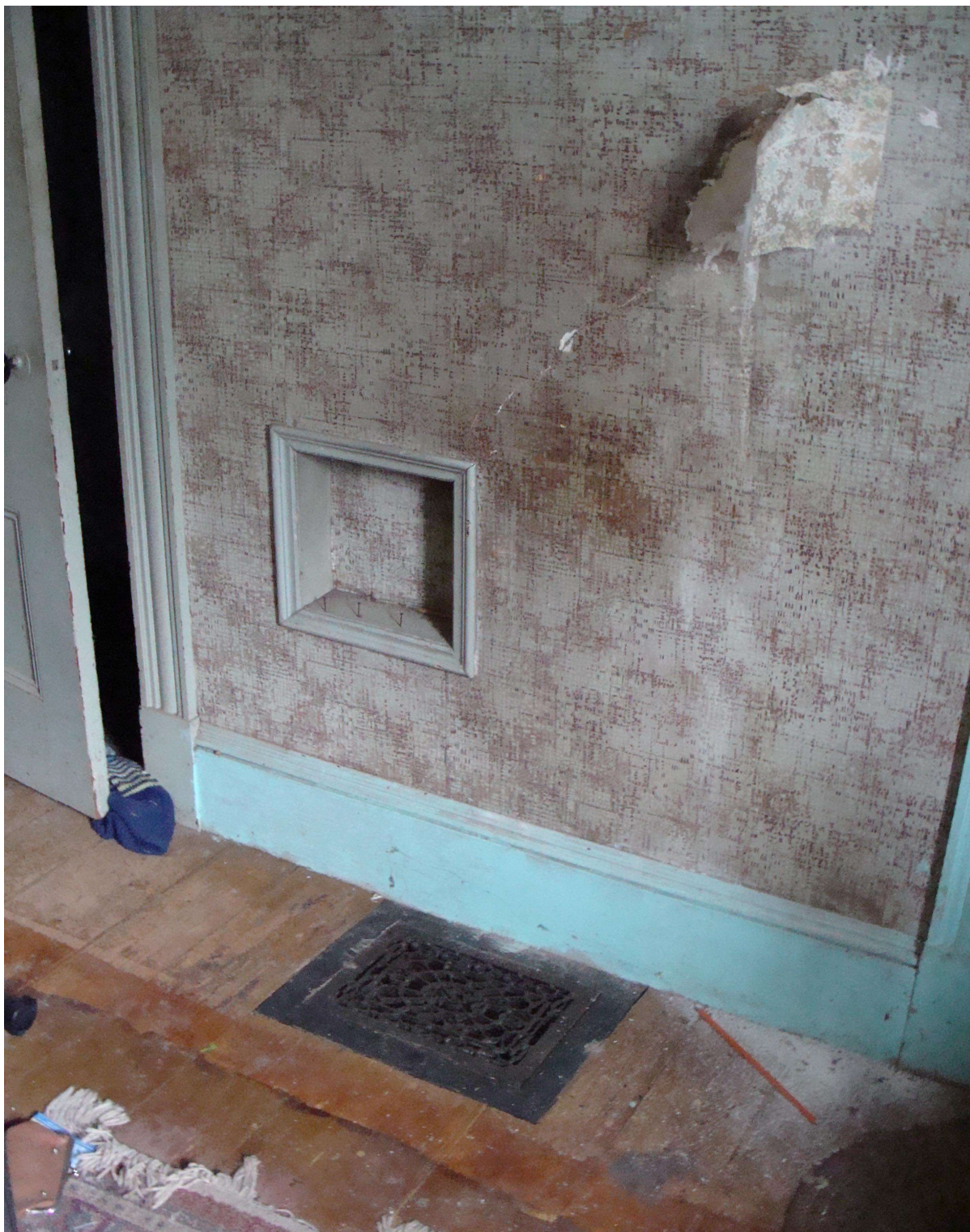
Figure 16. Detail, niche in the east wall of the parlor for a stove thimble. December 2015. Photograph by Myron O. Stachiw.
