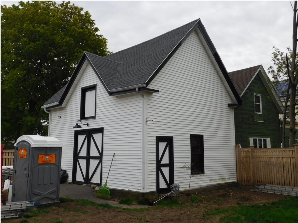
Carriage house from NE. Note early or original wood clapboard siding, doors and trim. The exterior light fixture above the main door is also an early surviving feature. The building appears to rest on wood sleepers.
