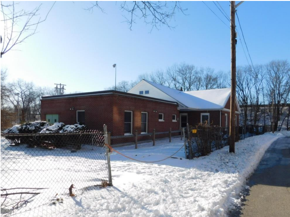
View from NE showing the 1991 wing, gable, and new second entrance.
