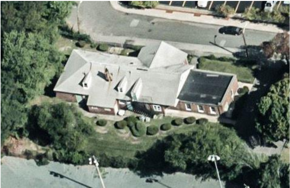
Aerial screen capture (Bing) facing N showing the rear elevation, dormers, and 2 nd -story egress.
