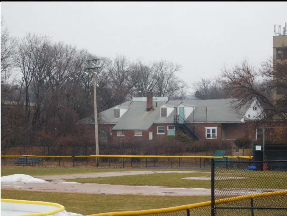
View from SE showing rear elevation.
