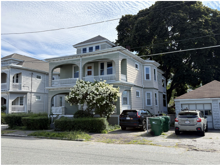
Two Family at 55 Surrey Street. The matching arched porch openings and surviving cornice details suggest original architectural treatments throughout the block.
